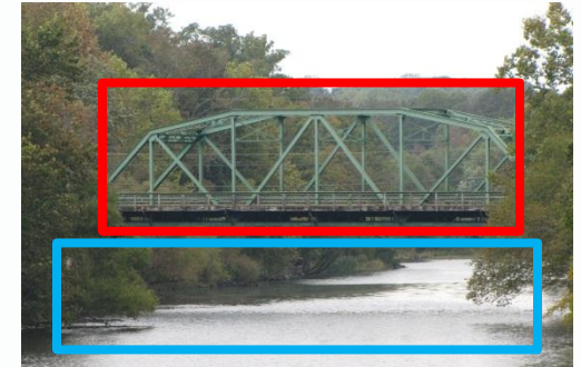
Iron bridge over the Duck river .
